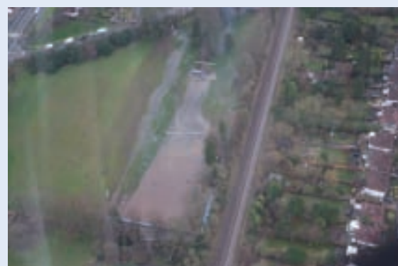
Aerial view of foul flooding in Bourne Park 14 th February 2014
