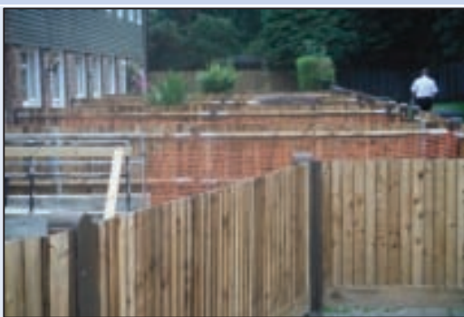
New fencing around gardens flooded by foul sewage in Bourne Park Close, July 2014
