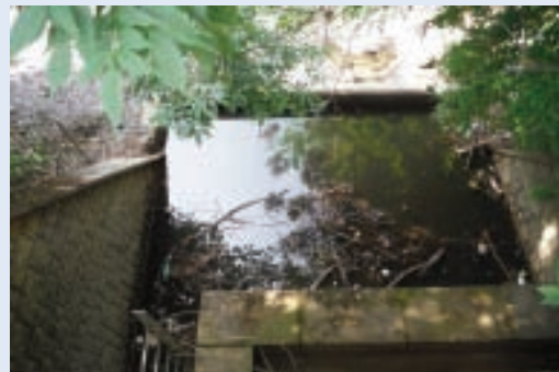
Sump area at north end of pond (July 2014)
