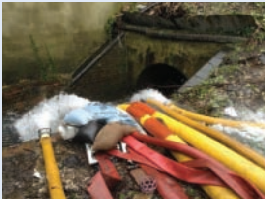
Water pumping into the bourne north of the railway line
