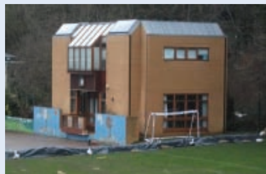
Temporary flood storage barriers set up around the school field
