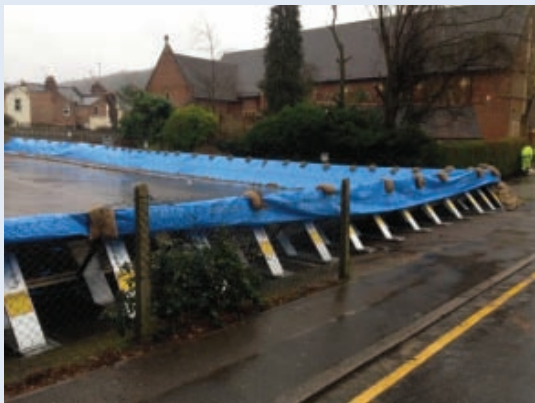
Church car park, emergency FSA
