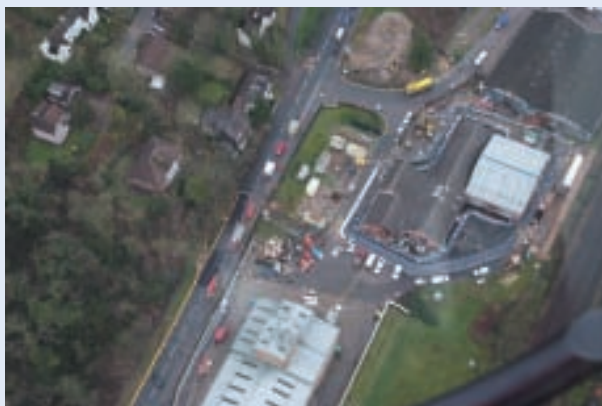
Aerial view of waterworks showing defences erected to protect infrastructure and pipes leading off down the A22 in February 2014
