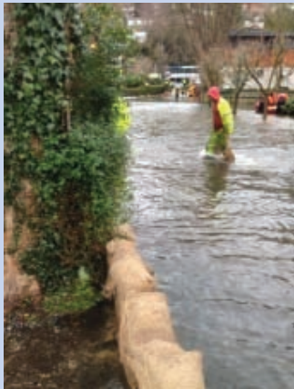
Response officers building sandbag walls in Dale Road in February 2014
