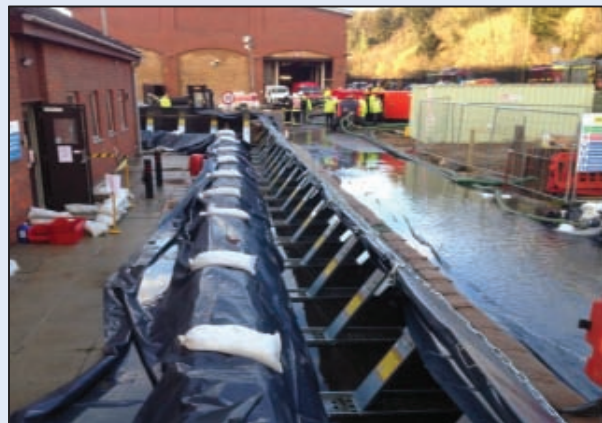
Demountable flood defences protecting the WTW
