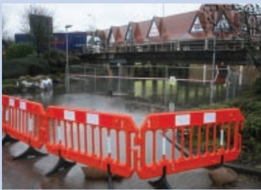
Inundation of the underpass at Purley Cross as a management measure to alleviate downstream flows towards Purley Oaks in February 2014
