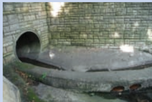
Culvert inlet to balancing pond after flood in July 2014
