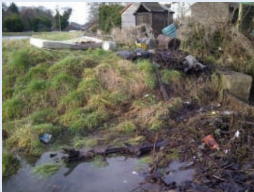
Fly tipping at Bourne View culvert on 18 th January 2014
