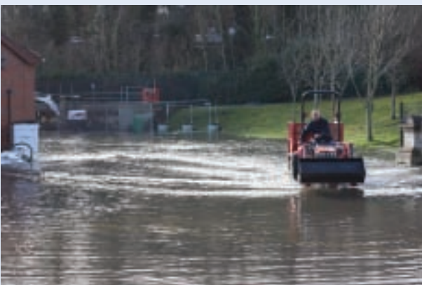
Floodwaters by main building at WTW in February 2014
