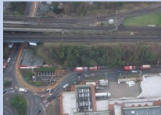
Water pumped from Dale Road and WTW around to an open section of the Bourne, north of the railway line in February 2014
