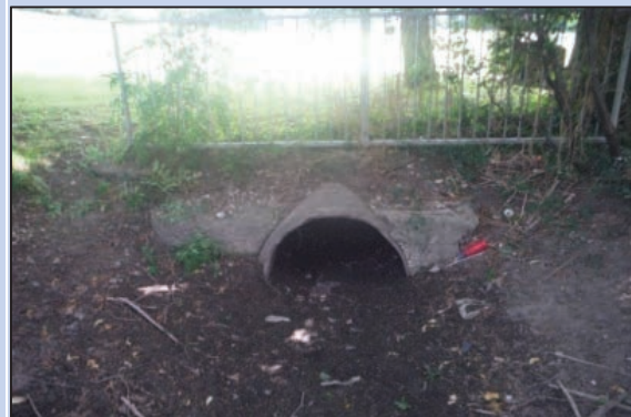
Silted culvert in Bourne Park following flood, July 2014
