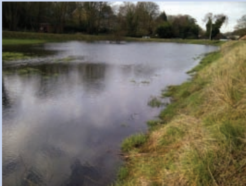
Bourne View flood storage area already filling up on January 18 th 2014
