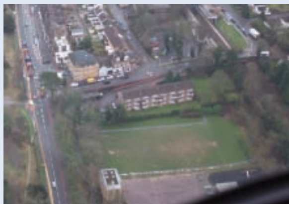
Temporary flood storage barriers set up around the school field
