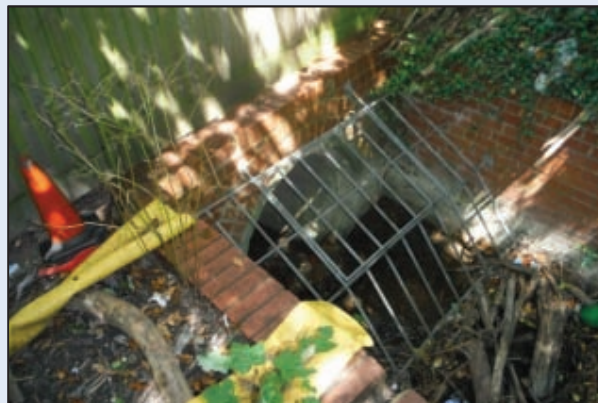
Culvert and Trash Screen downstream of Cricket Ground in January 2014
