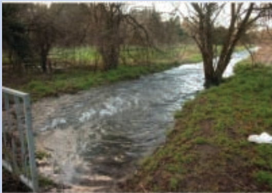
Open section of bourne flowing NW out of culvert at Bourne Park, February 2014
