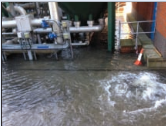
Surcharging bourne culvert
