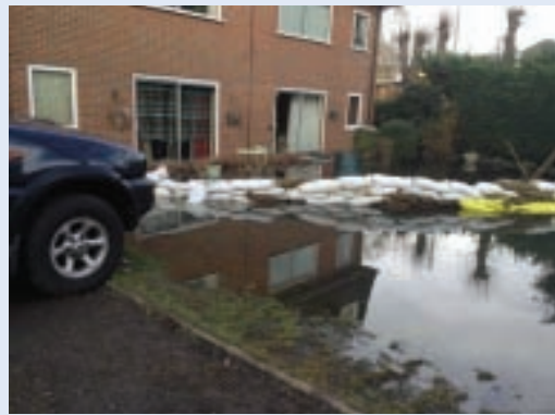
Flooding at rear of Liddell Court on Foxley Hill Road, February 2014
